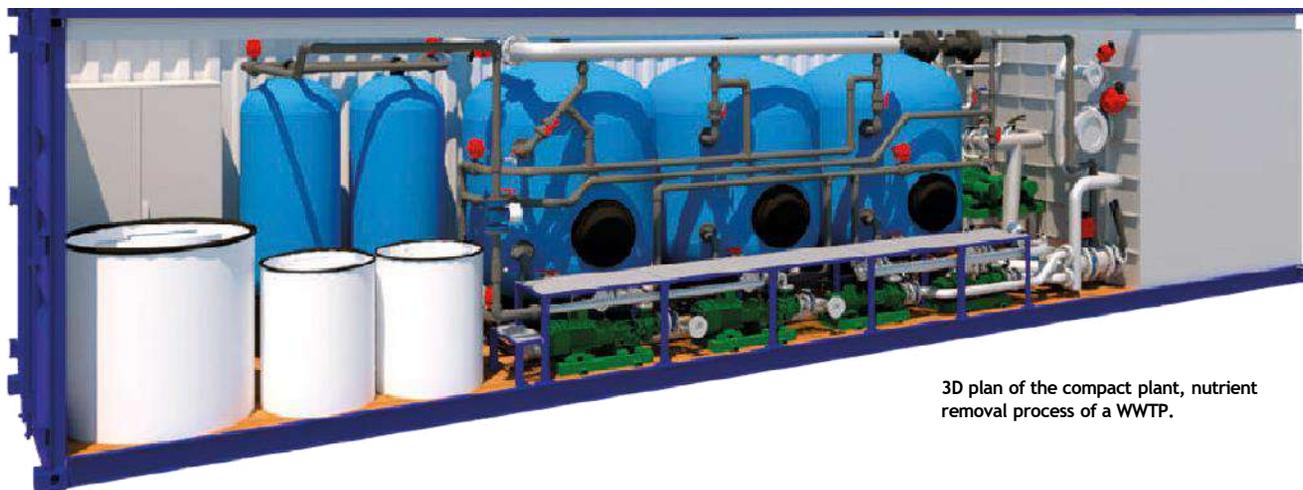
3D plan of the compact plant, nutrient removal process of a WWTP.
