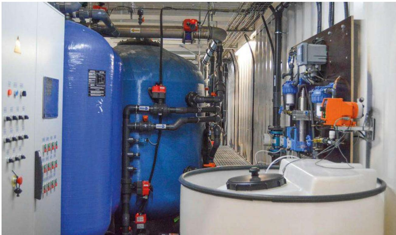
Image of the interior of a compact plant, nutrient removal process of a WWTP.
